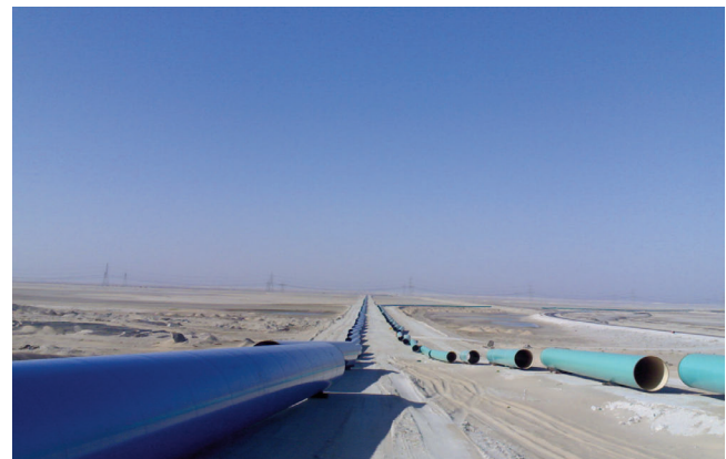
Figure 11. Pipeline Sections Ready for Welding in Saudi Arabia.
