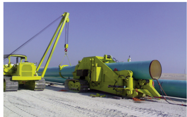
Figure 12. Pipeline Bending Process.
