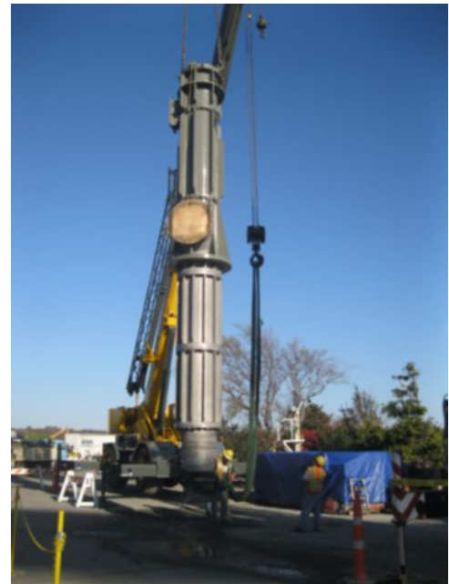
Service Water Pump
