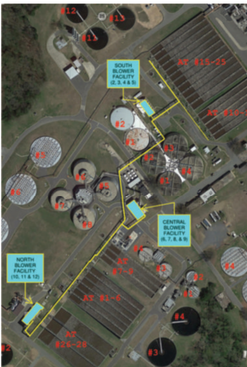
Figure 1: The original aeration system which included three blower facilities with a total of 11 blowers that provide air to 28 aeration tanks around the plant. The yellow lines on the map show the air manifold connecting all of the air piping and blower facilities.
